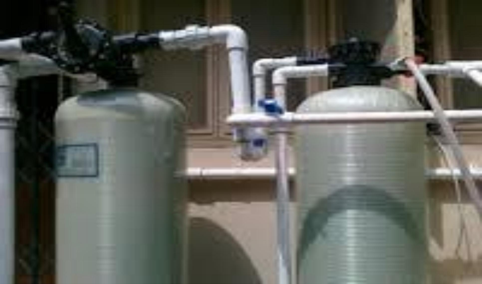
**Activated CARBON filter on your pool water make up line. Remove chloramines from city water.**
